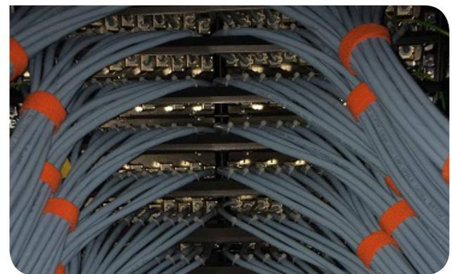
patch cords. Excel Category 6<sub>A</sub> Harness links were also built specifically for Cisco Nexus switches, reducing the overall cost of the project so that multiple adjacent racks could share the same backbone switching fabric and DMZ security requirements.
